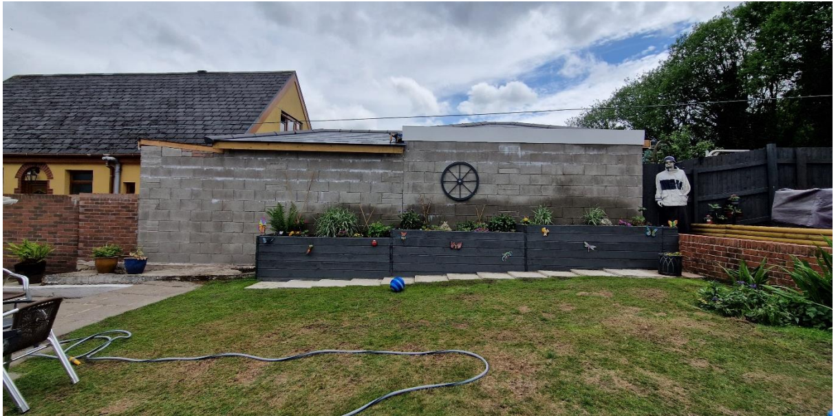
Figure 1.8 Photo showing views from existing balcony are now obscured due to intervening outbuilding
