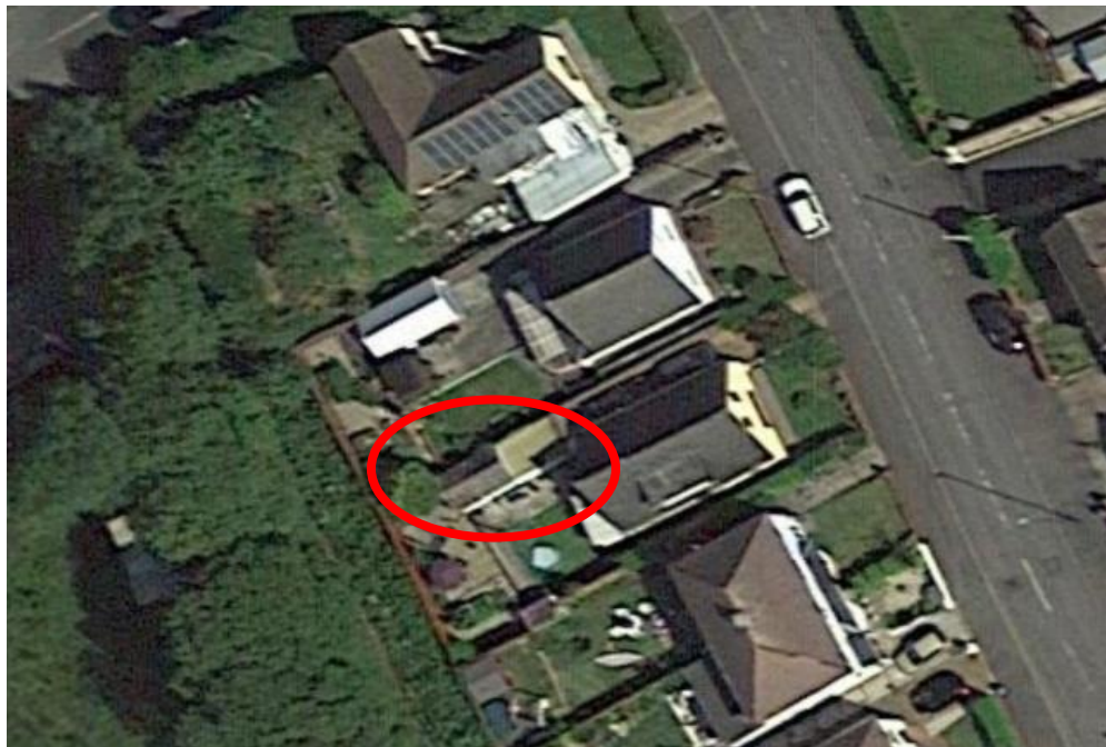
Figure 1.10 Aerial image of site from 2021 showing location of pre-existing garage and outbuilding
